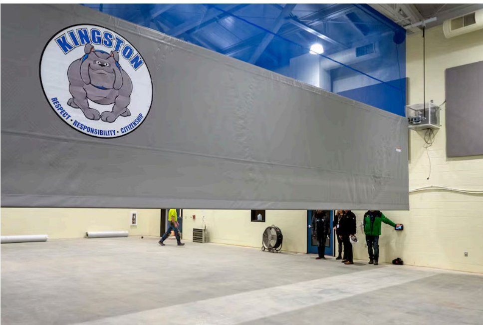
Cherry Hill School District director of facilities Steve Nicolella (hidden) demonstrates the lowering of the panel screen to divide the almost completed new all-purpose room and gym at Kingston Elem Read more
