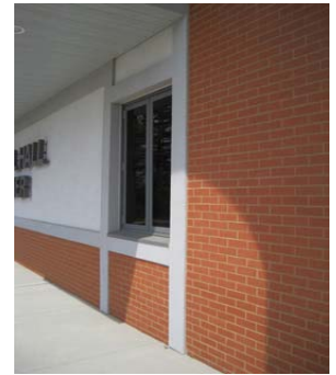
“Thin Brick” Exterior Wall
