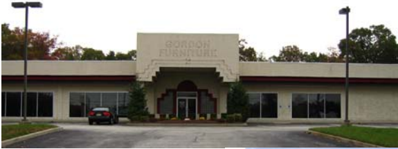
◀ BEFORE: An abandoned retail store prominently on Route 73, vacant and deteriorating.
